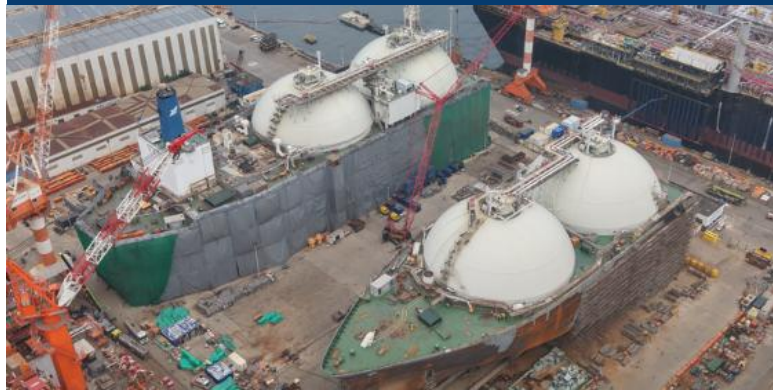
Donor vessel cut – repairs and upgrades ongoing
