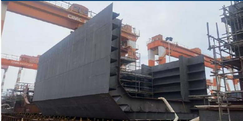
Sponson fabrication ongoing
